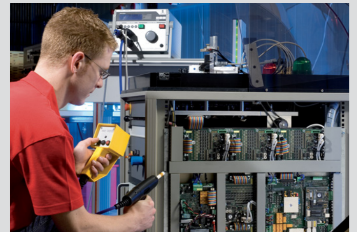
EN60204 test at a service cabinet
